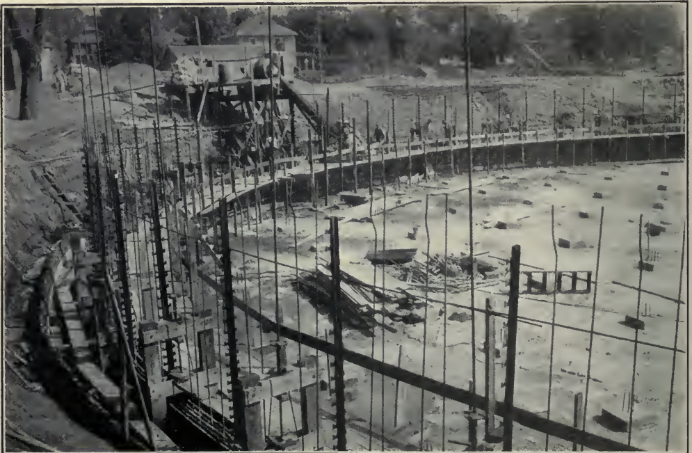
CONSTRUCTING RESERVOIR WALL, USING THE SLIP FORM METHOD
